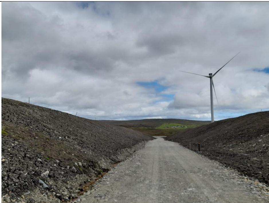
Photo 17. Reprofilng and hydroseeding of embankment at Spur 52 in North Nesting
