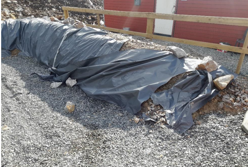
Photo 3. Sheeting in poor condition within refuelling bund in Vestas Compound
