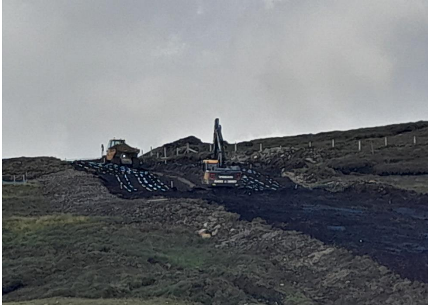
Photo 9. Cable trench backfilling on the cross-country route from mid Kames Ridge to Sandwater Road
