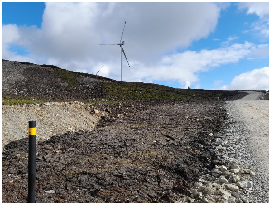
Photo 1. Backfilling cables in Kergord Area
