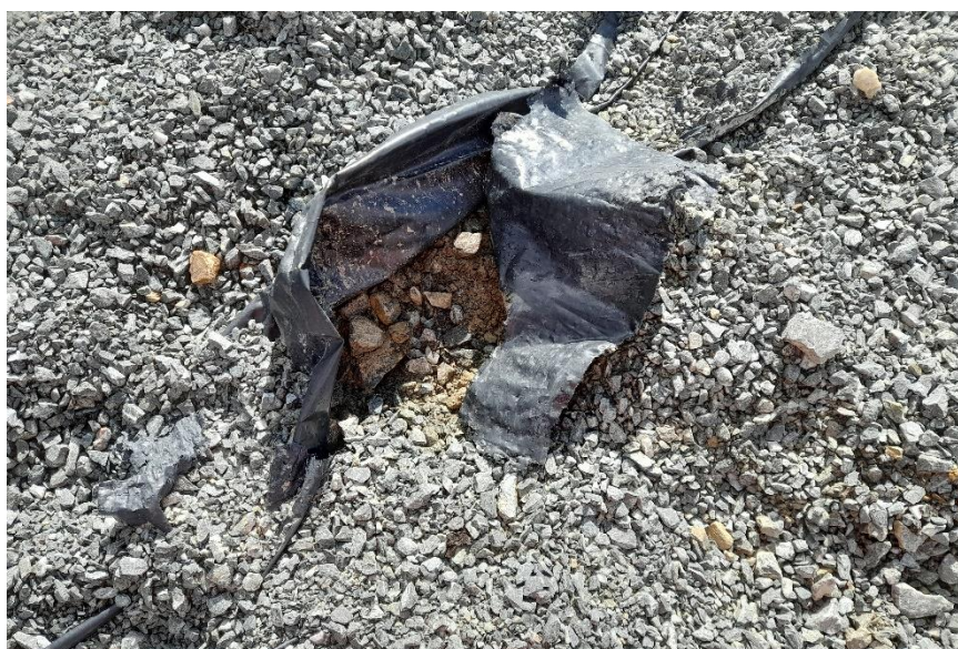
Photo 2. Sheetting in poor condition within refuelling bund in Vestas Compound
