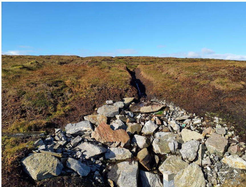
Photo 7. Upgraded drainage by T001, view upstream of track with swale
