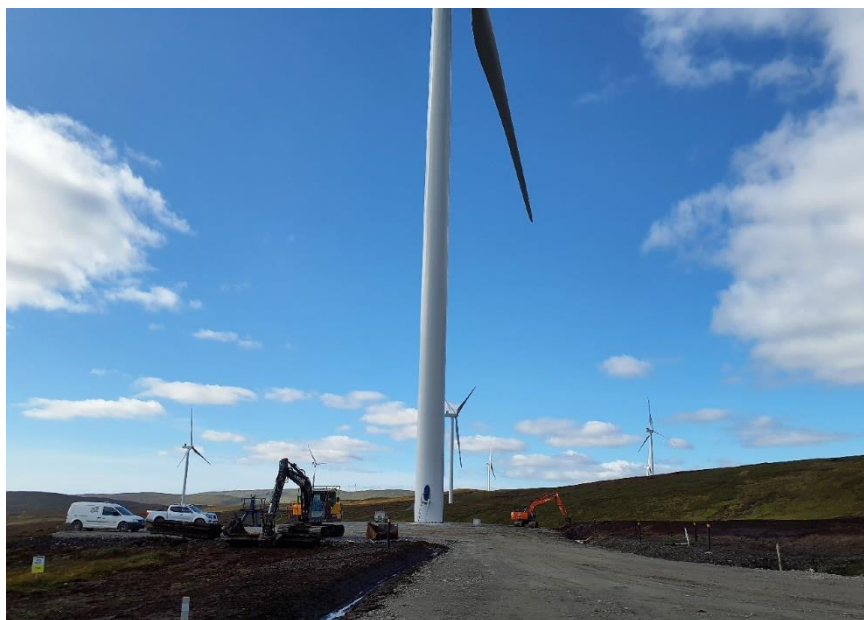
Photo 14. Active turbine hardstand reinstatement by T100
