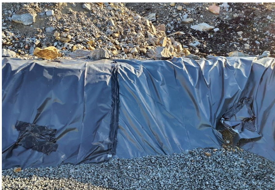
Photo 2. Taped sheeting with remaining tear within refuelling bund in Vestas Compound
