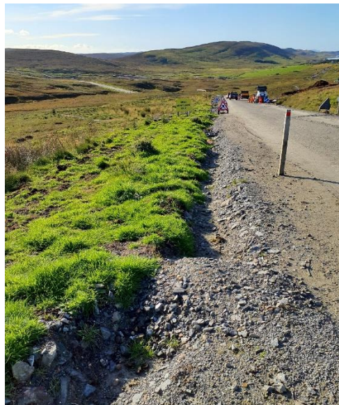
Photo 10. Check dams in trackside drainage at the junction between KAT and Spur 5
