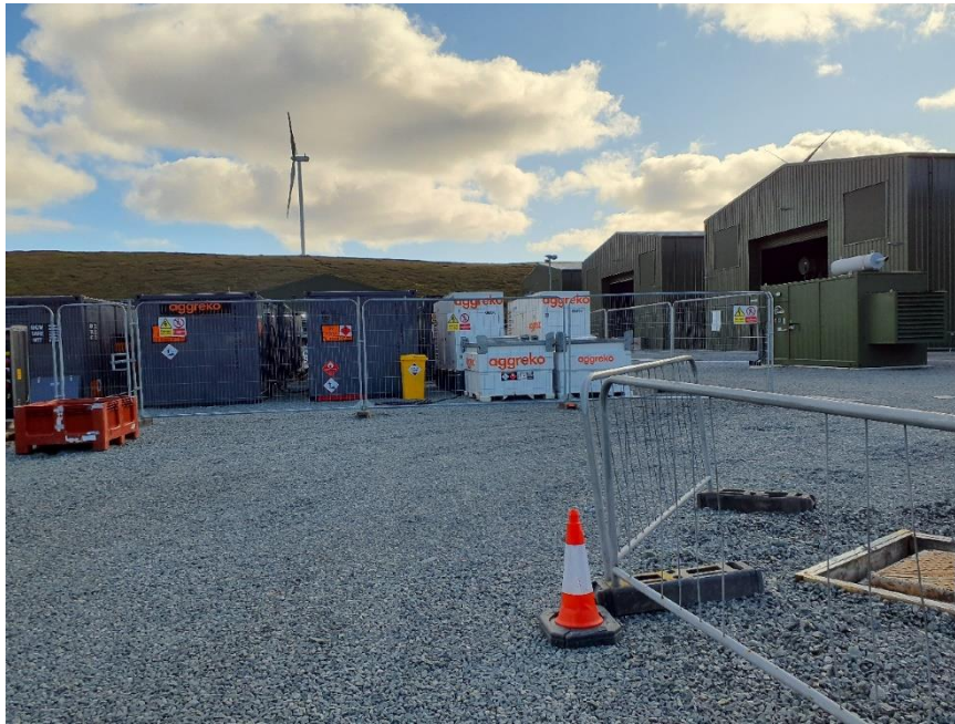
Photo 17. Aggreko Commissioning Generator Package Set-Up
