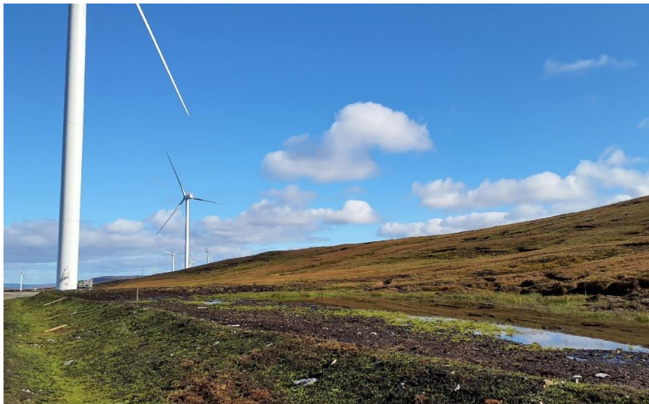
Photo 6. Reinstated track and turbine hardstand with road-side pond by T004
