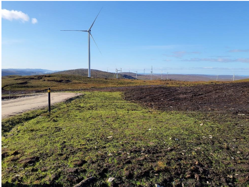
Photo 1. Hydroseeding on backfilled cable trenches near T021
