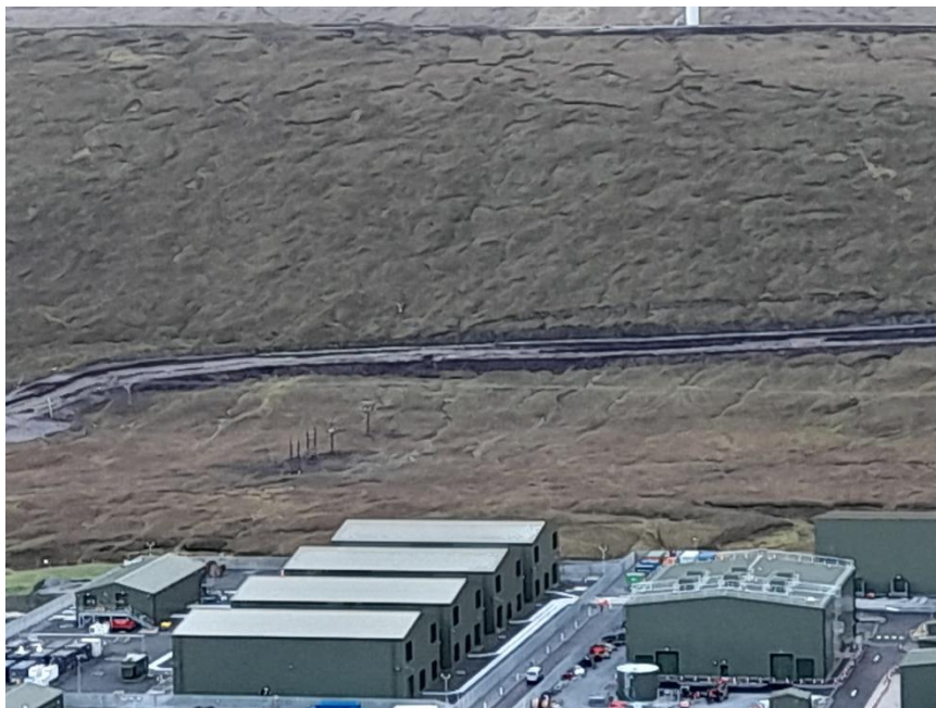
Photo 8. Repair of bund on the Mid Kames Ridge to substation cross country track and installation of silt fences following a silty water event in the Burn of Weisdale
