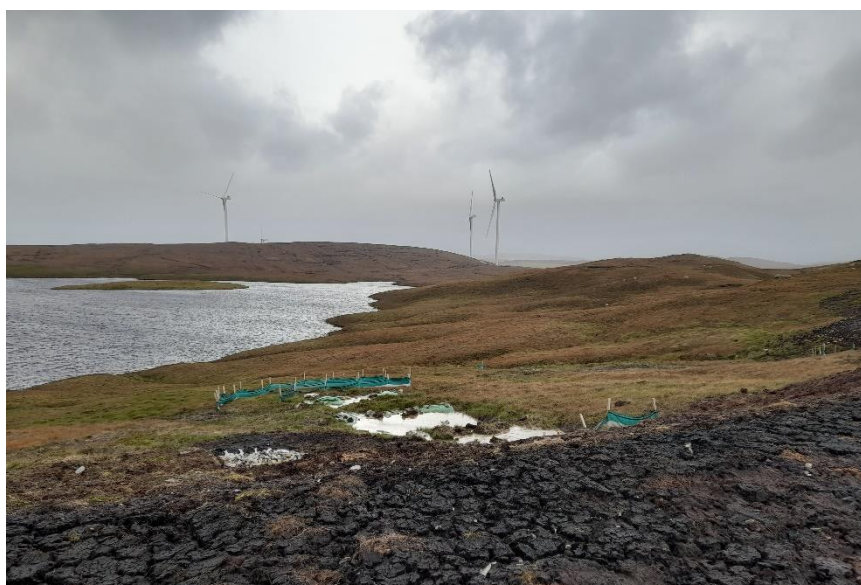
Photo 6. Settlement ponds for diverted water from KBP03 at Maa Loch
