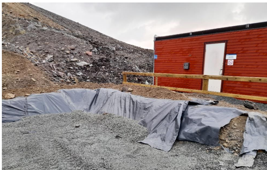
Photo 3. Breaches in refuelling bund in KBP05 being repaired
