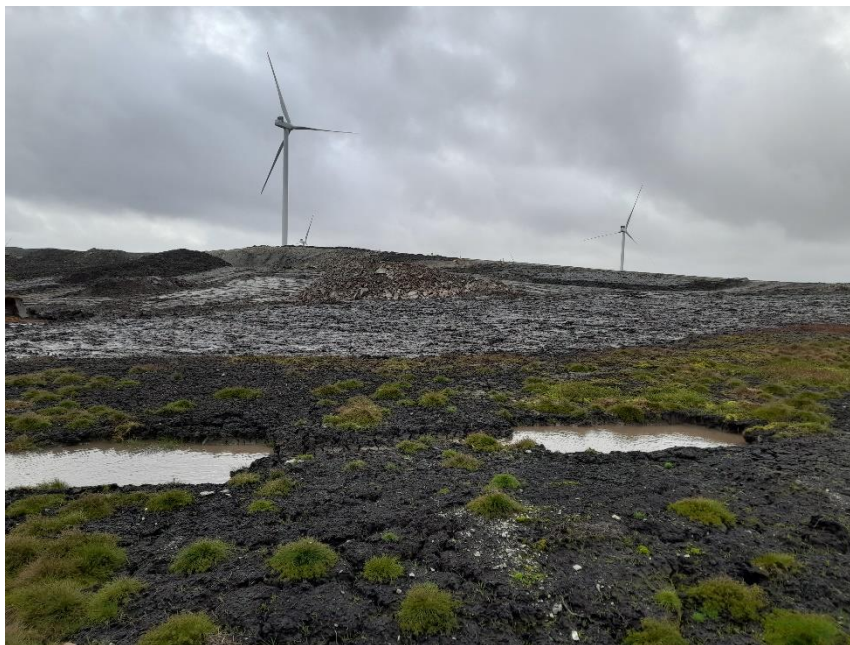
Photo 16. Settlement ponds installed at NBP05
