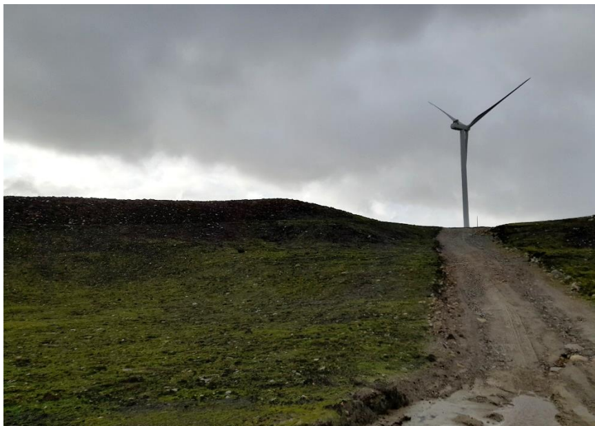
Photo 2. Reprofilling and hydroseeding in KBP02
