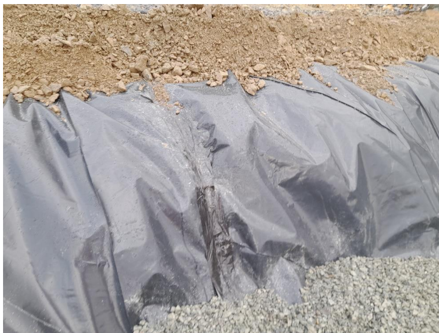
Photo 4. Repair of lining in refuelling bund in KBP05
