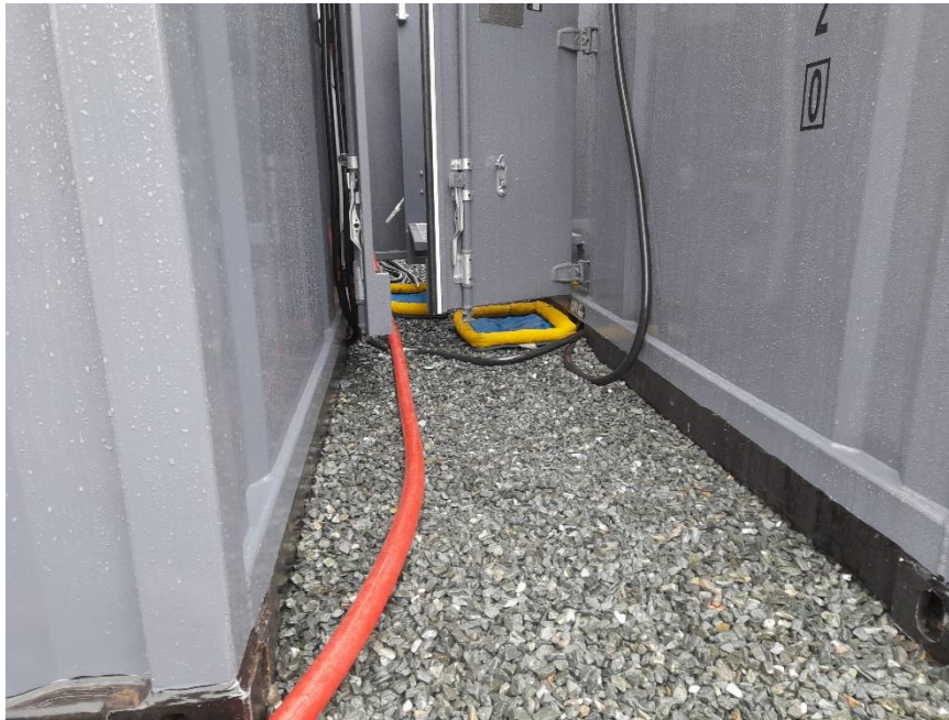
Photo 17. Drip trays / plant nappies in place during the refuelling of generators in the substation
