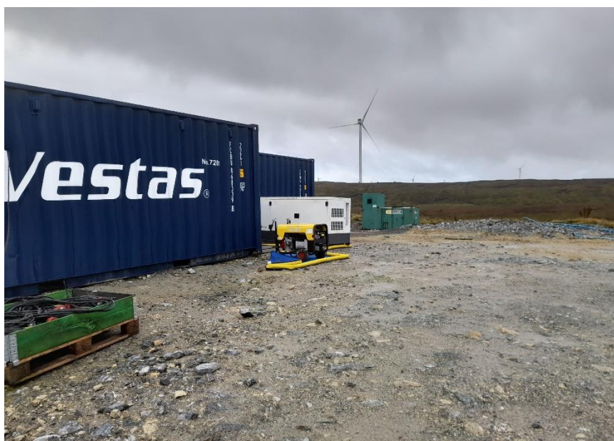
Photo 12. Plant nappies beneath generators in northern compound
