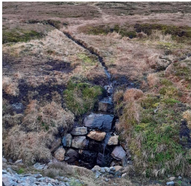
Photo 14. Permanent drainage good practice at T099
