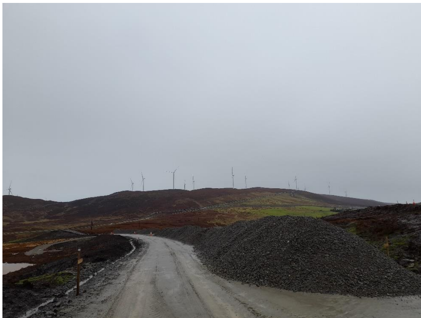
Photo 6. Material from borrow pits being used to raise the Sandwater track.
