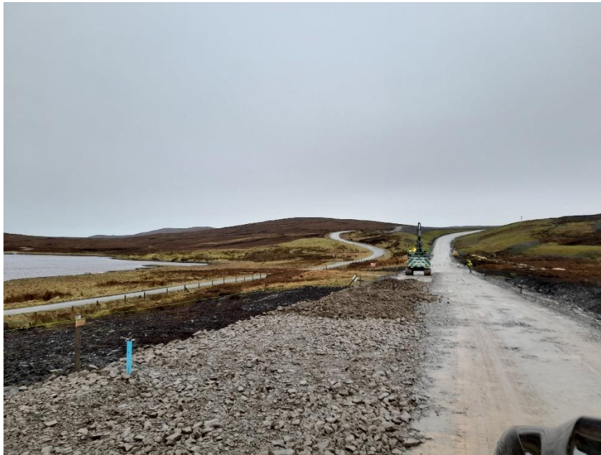
Photo 5. Raising the Sandwater track.
